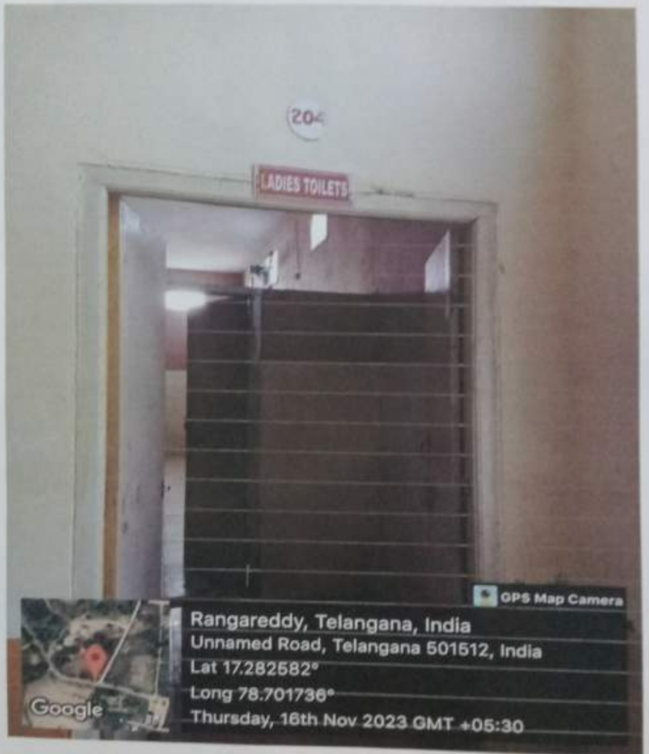
Seperate washroom facility for women
