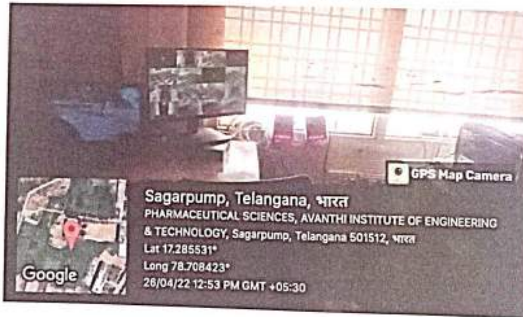
Ce Surveillance with router in principal Room, Ground floor
